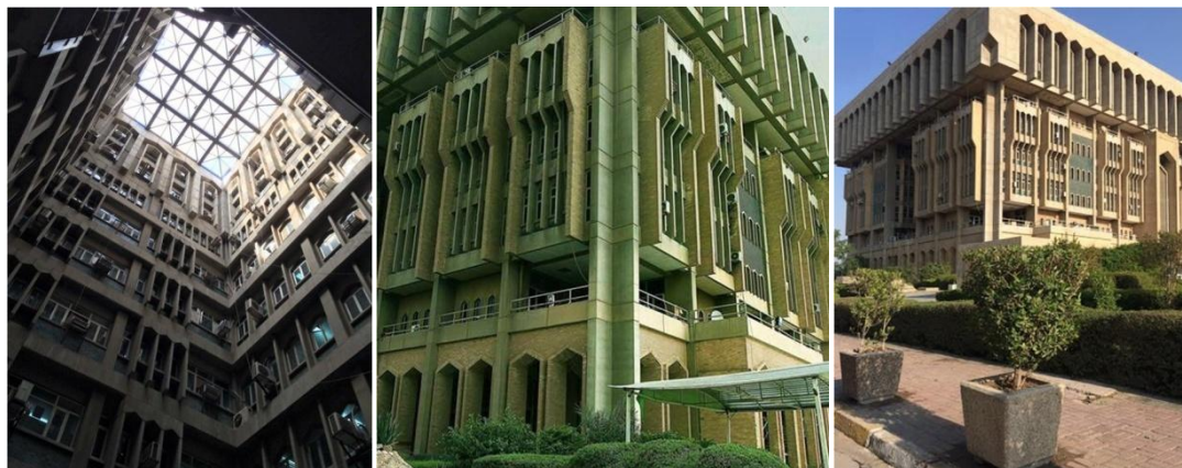
Figure 14: Treatment of external facades, reducing the effect of direct solar radiation, and the internal ventilation system. (By the researcher)
