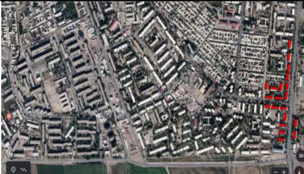
Figure 3. Aerial view of panel residential buildings in Kirguli region of Fergana city.
