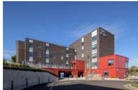
Figure 6: The colorful vertical fin façade helps to 'bring together' the new and old elements of the building [26].
