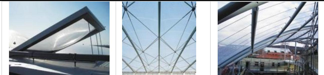
The building structures implemented with the help of ETFE can be single-layer and multilayer. In addition to roofs and facades of buildings, with the help of single-layer film structures, it can be organized any non-standard objects, all kinds of canopies, umbrellas. Multilayer systems consist of pneumatic membrane cushions enclosed in
