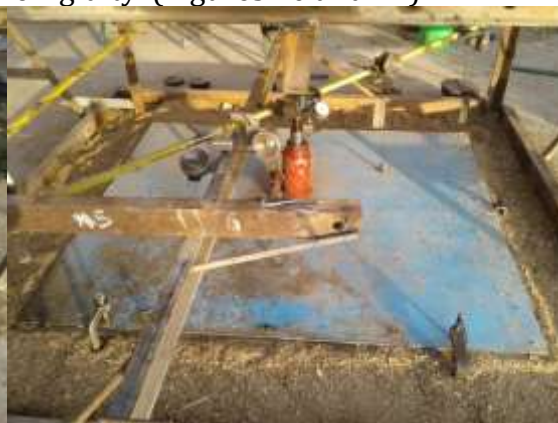
Figure 11. Installation of the metal plate with tripled rigidity.
