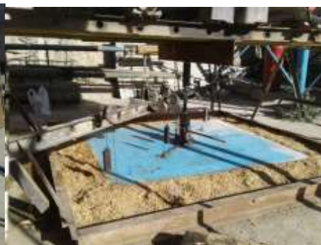
Figure 2. Installation of a hydraulic jack.
