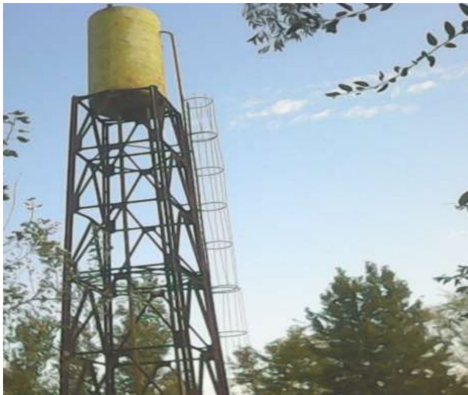
Fig. 3 - Geothermal borehole tower of the sanatorium "Altyaryk".
