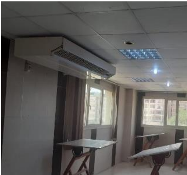
Figure 8: Using ceramic to finish interior walls
