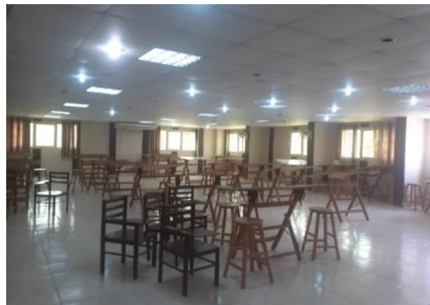
Figure 12: Using inappropriate lighting in classrooms
