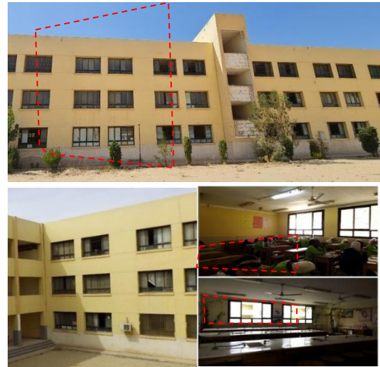
Figure (6): shows the students' use of screens and curtains on the windows to protect against glare and solar radiation inside the classroom, which blocks natural lighting inside the space. Source: researcher
