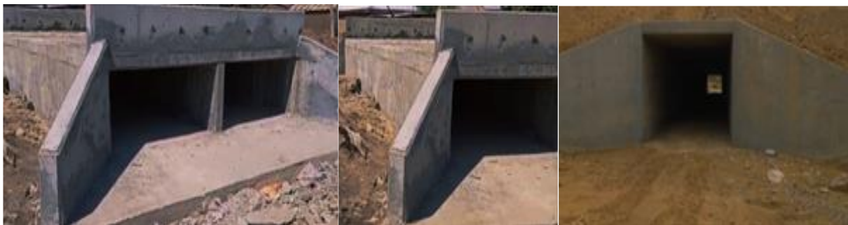
Figure 12. Some forms of Box Culverts
