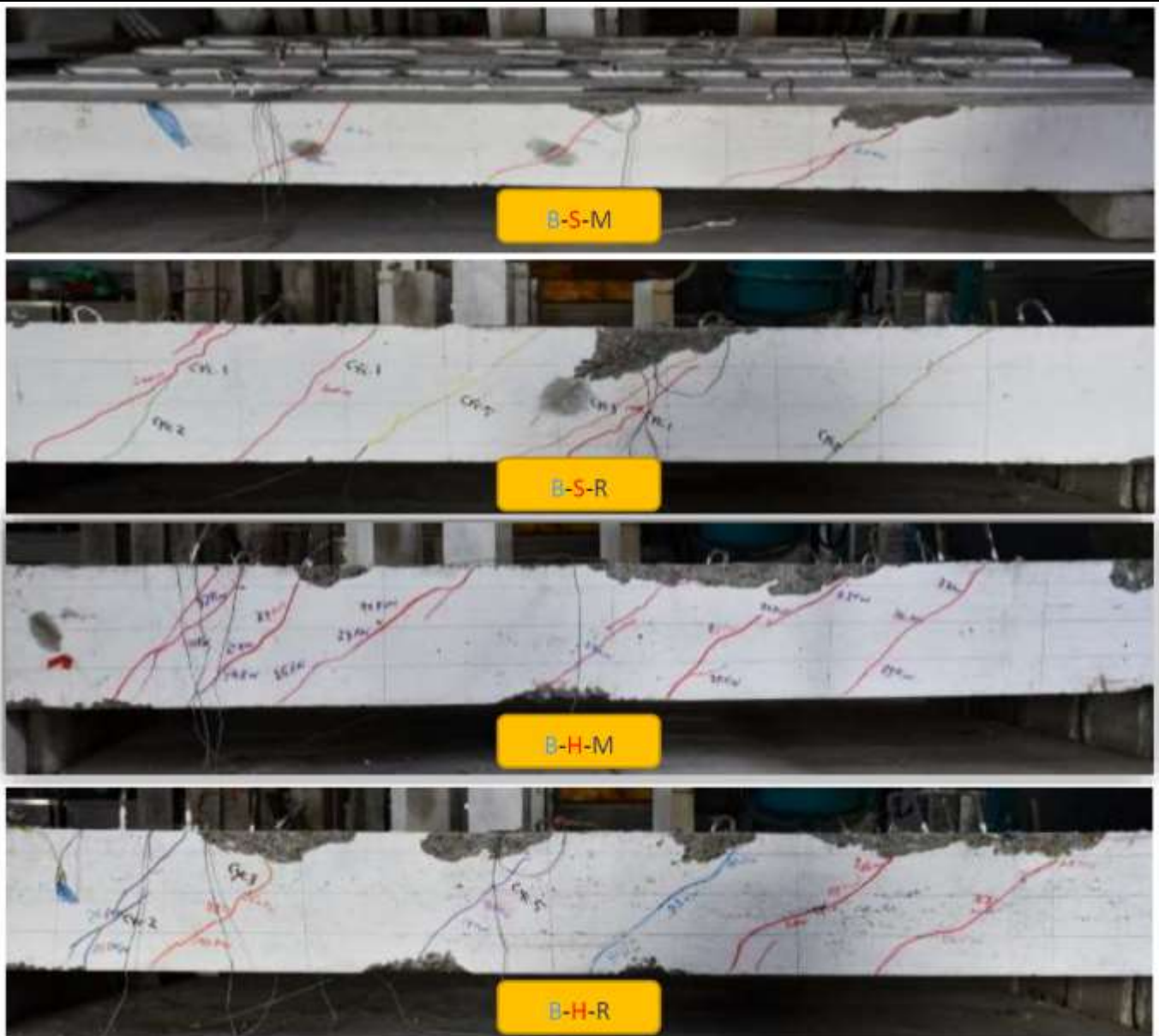
Figure 20: Failure modes of beams tested under monotonic and repeated loads.
