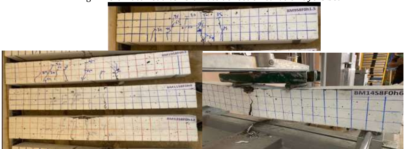
Figure (23) : Cracks Pattern of SFRCH (beam layers
