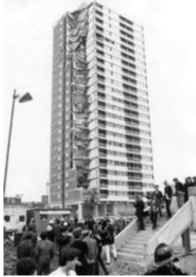
Figure 2: The Ronan Point apartment partial collapse [Nair, (2004)].
