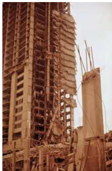
Figure 3: Progressive collapse of Skyline Tower [Schellhammer et al.,(2013)].
