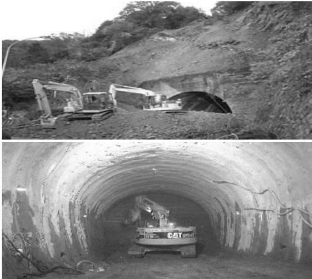
Fig. 1 Excavator work under bad environment
