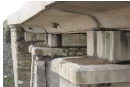
Figure 5. Span - slab, reinforced concrete
