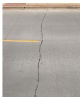
Transverse and diagonal cracks Regardless of orientation, these types of cracks differ from mapping cracks or other surface cracks in that they are distinct cracks that typically run through the entire thickness of the slab.
